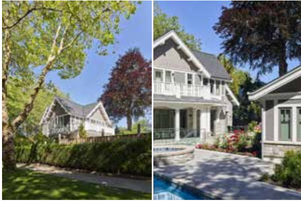
A resistance pool with a hot tub is placed on the south side for sun exposure to extend the usable season. Both the hot tub and the pool has their own in-ground automatic covers which are utilized when not in use for energy-saving and safety. Pool users have quick access to the change/shower area in the garden room next to the garage. The planting area is strategically positioned at side yards, in front of the garage/garden room and
